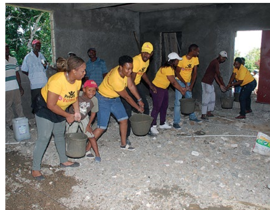
Team Work! Victoria Mutual Volunteers doing construction work.
